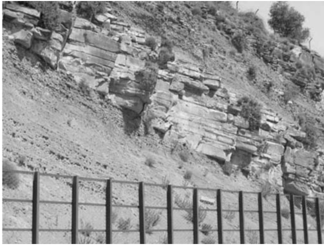
Fig. 8: Alternated layers of sandstones and siltstones of flysch formation (Evinochori region).
